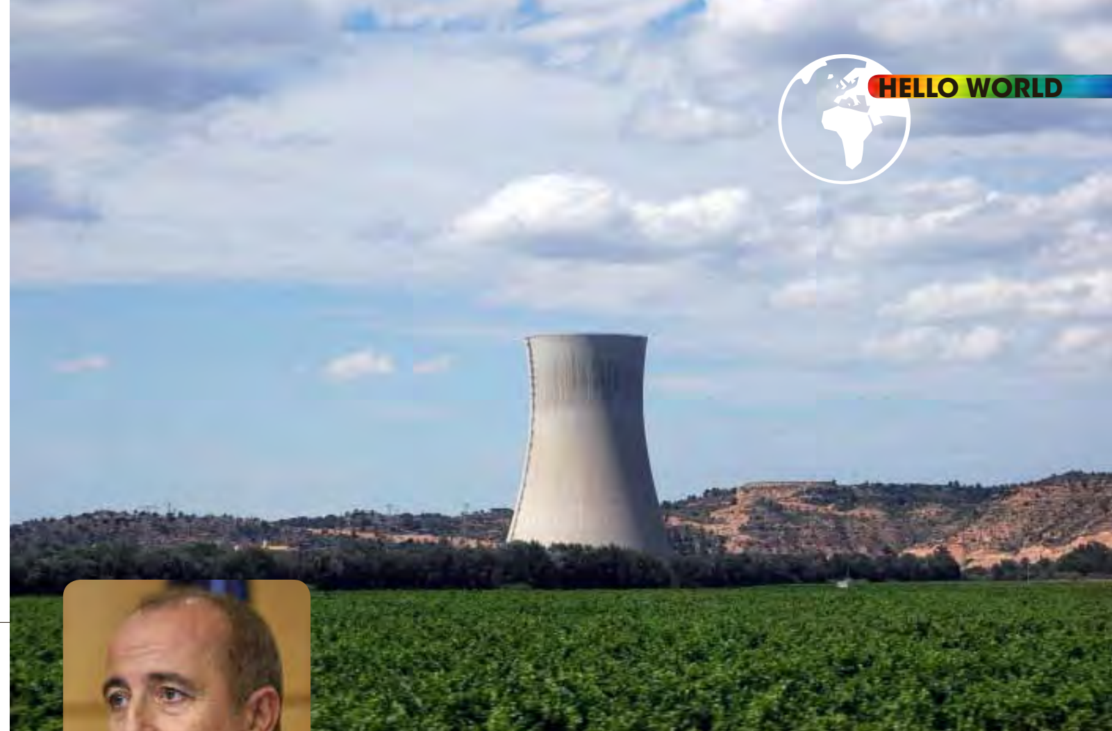
Picture from Ascó Nuclear Power Plant. Spain has eight nuclear reactors generating a fifth of its electricity. Its first commercial nuclear power reactor began operating in 1968.
